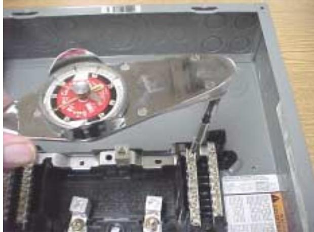
**Figure 10:** Torque new neutral plate screws
