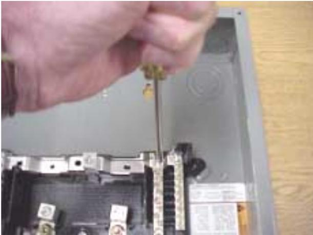
**Figure 9:** Install new neutral plate screws.
