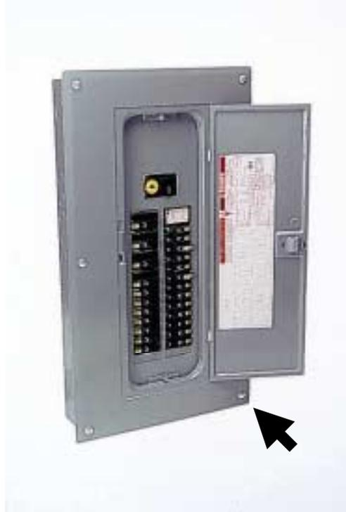
**Figure 4:** Typical QO Main Breaker Load Centre – Catalog Number CQOxxxxxx
