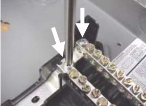
Figure 7: Locate neutral plate screws
