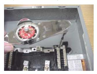
Figure 9: Install new neutral plate screws.
